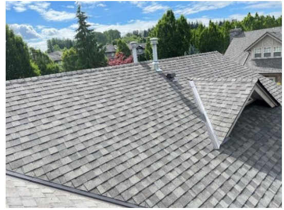
View of completed new asphalt shingle assembly at a sloped roof.
